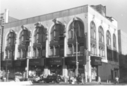
(Former) Hamilton Theatre, 3560-3568 Broadway, Manhattan. Built 1912-13; Architect Thomas W. Lamb-courtesy New York City Landmarks Commission
